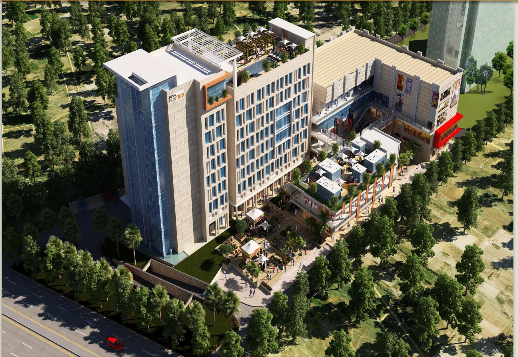
Project View - Front
